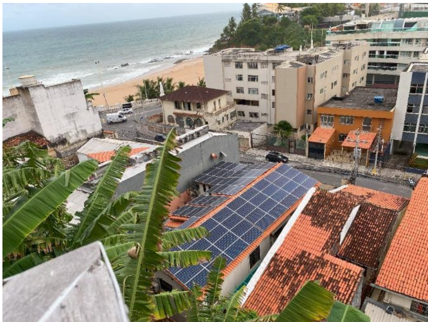
Solar panels, Salvador, Brazil
